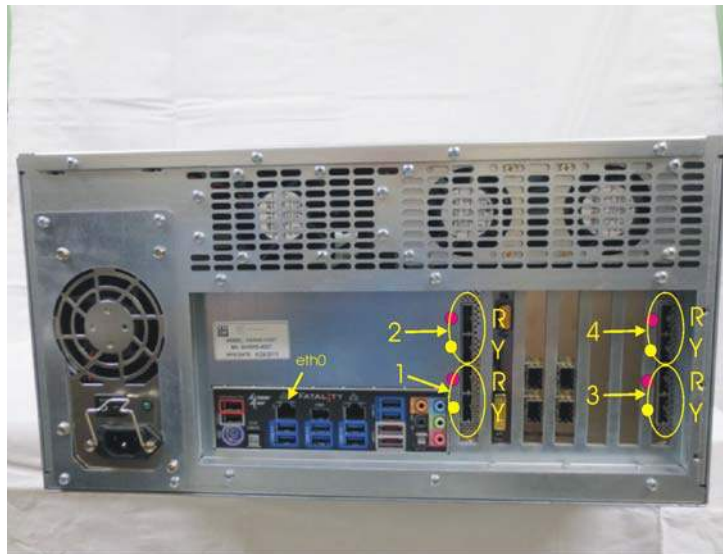
Figure 2: mini-SAS cable connections to host-bus adapter (i.e. disk interface) cards on rear of system chassis. Numbers correspond to cable tray labeling. 'R' is for red-labeled cables, 'Y' for yellow-labeled cables. Positions '3' and '4' will not be used (and may not exist) if an expansion chassis is not installed. Position of 'eth0' network connector is also shown.
